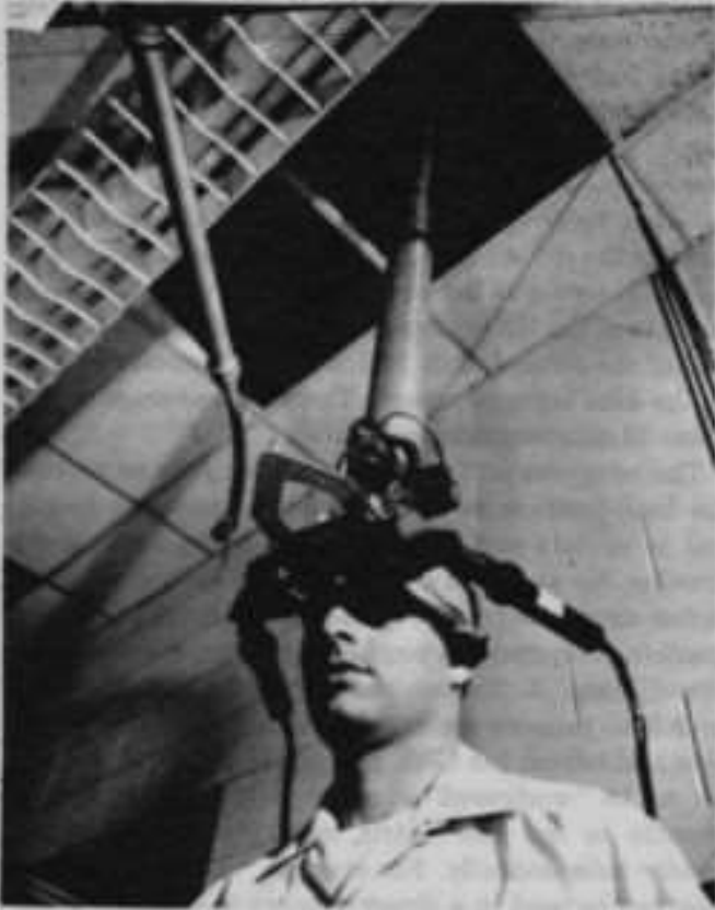
FIGURE 4--The ultrasonic head position sensor in use
